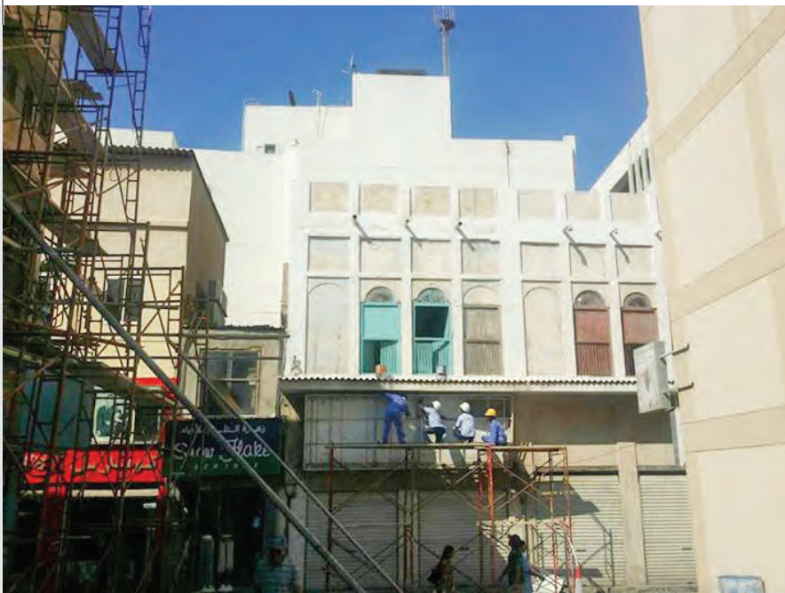
Painting and decoration works in progress.
