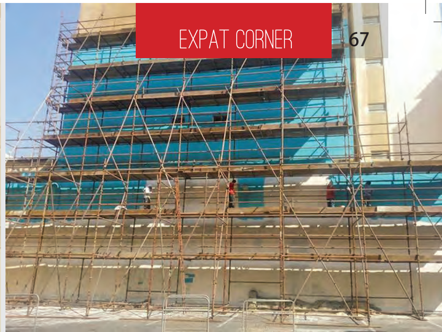
Buildings being painted.
