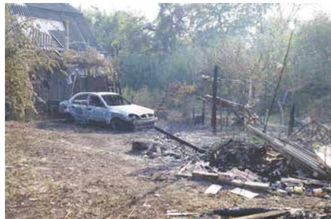
A burned car and a damaged residential building following a Russian air attack in the Kyiv region
