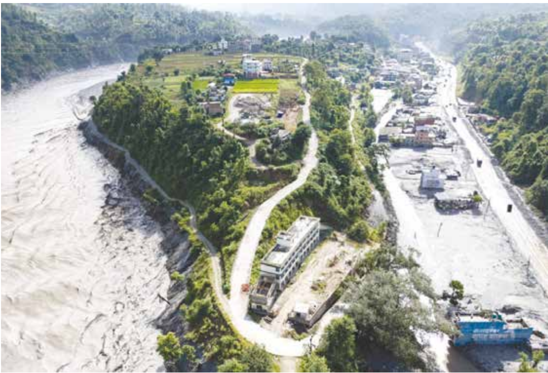
An overflowing Trishuli River (L) and houses covered in mud (R) in the aftermath of flash floods at Baireni in Nepal's Dhading district
