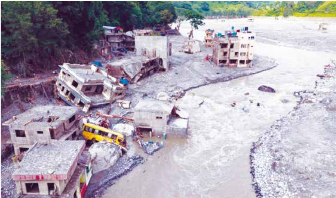
A torrent of muddy water surging past houses and through the Trishuli river in the aftermath of flash floods, at Betrawati in Nepal's Nuwakot district
