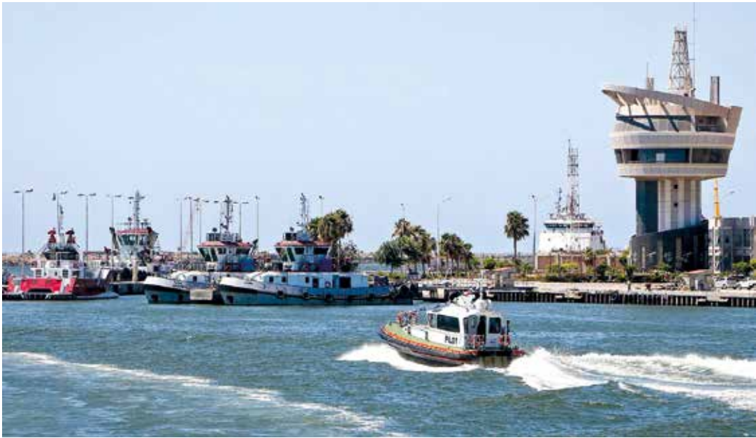
A view of the control tower of the Mediterranean sea port of Damietta in Egypt
