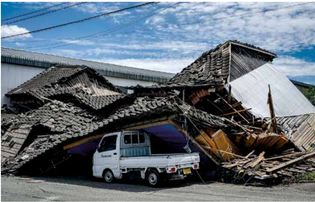
A house is seen collapsed onto a car in Yatsushiro, Kumamoto prefecture
