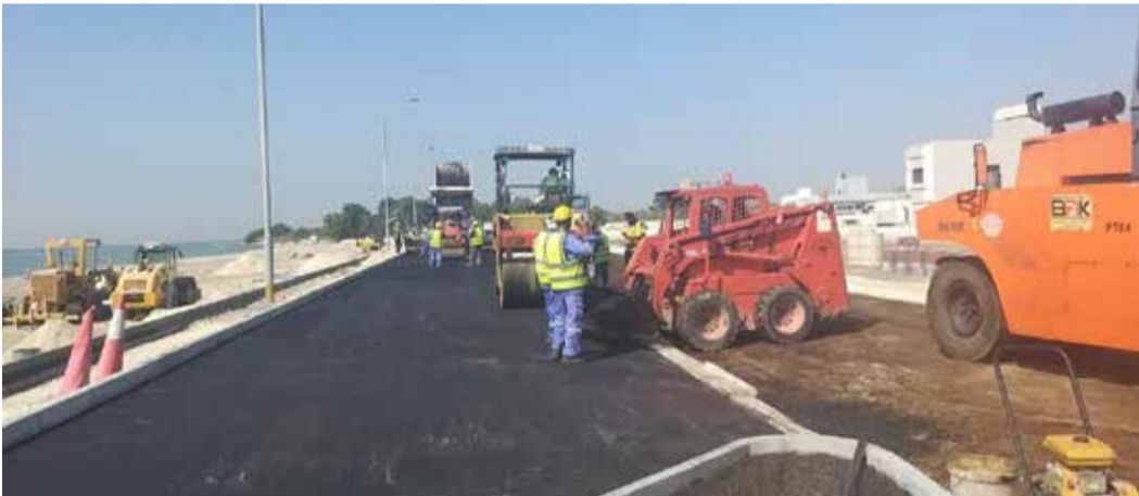
Road work in progress
