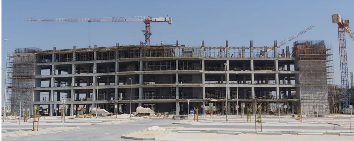
Works at the site in progress
