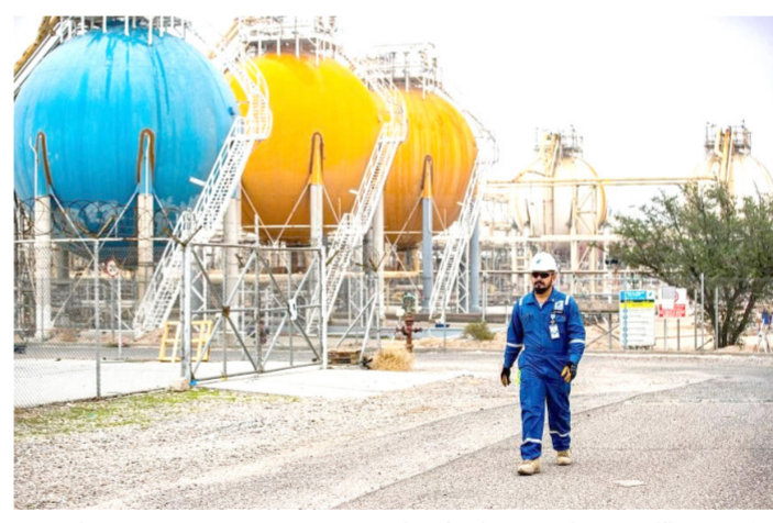
An engineer walks past tanks at the gas liquefaction plant in Basra (file photo)
