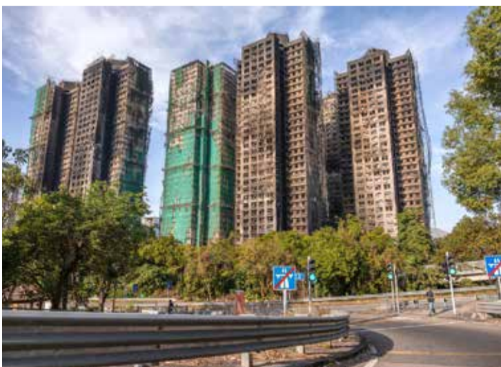
A general view shows the aftermath of a major fire that swept through several apartment blocks at the Wang Fuk Court residential estate in Hong Kong
