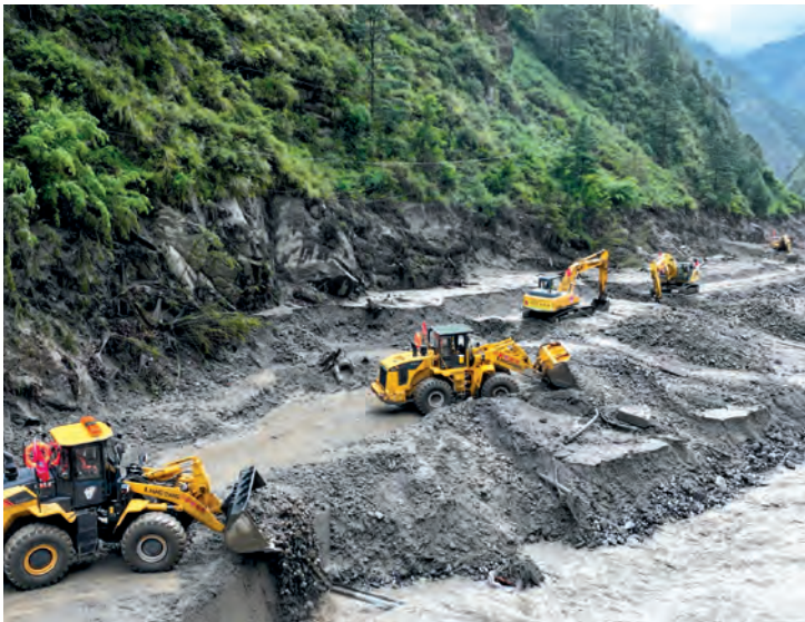
Workers repair a section of road leading to Gyirong Port which was damaged after a mudslide two days earlier, in Gyirong County, in China’s western Tibet region
