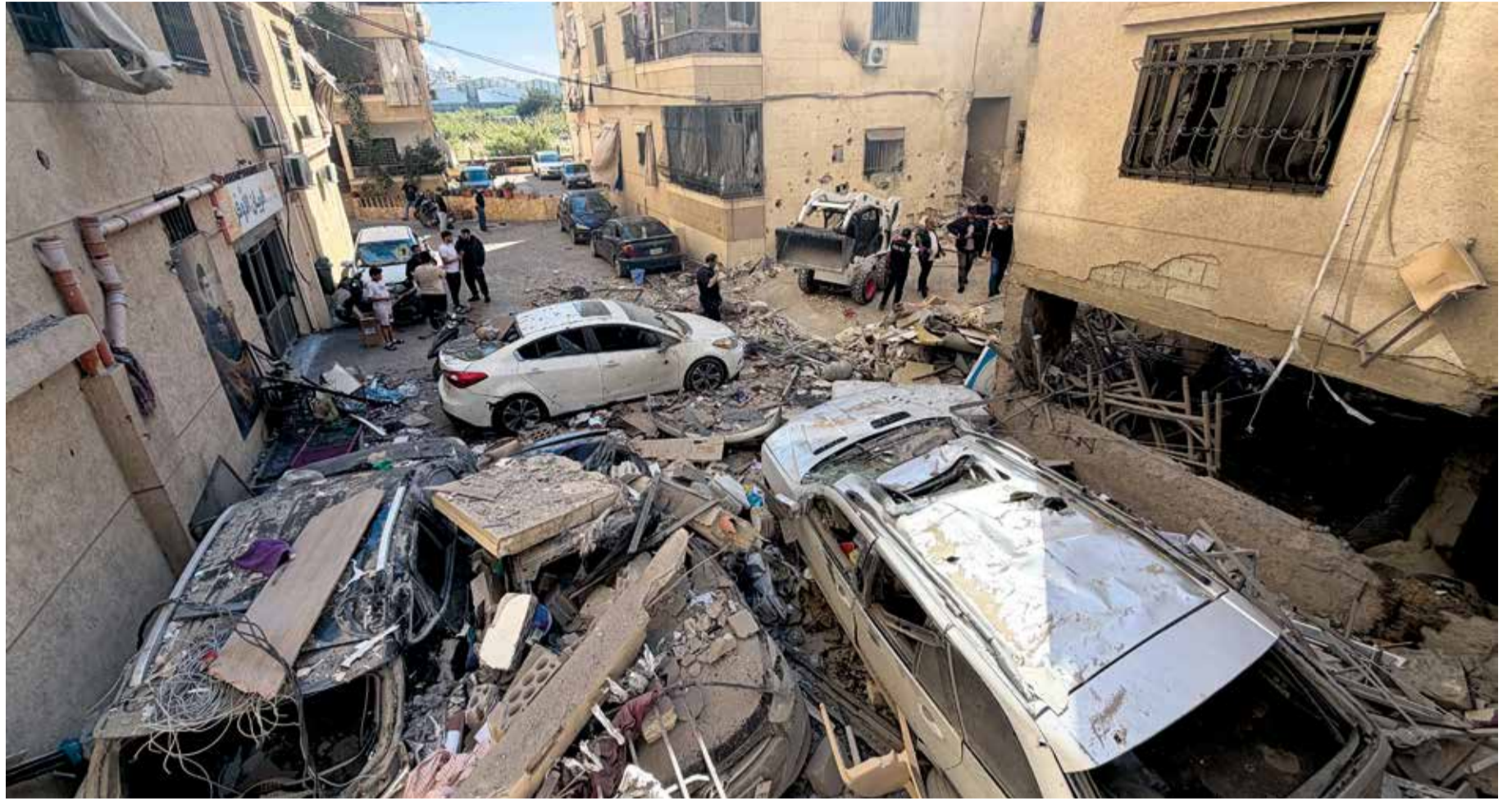
Rescue workers and local residents inspect the damage to a building following an Israeli air strike in the Choueifat area, south of Beirut
