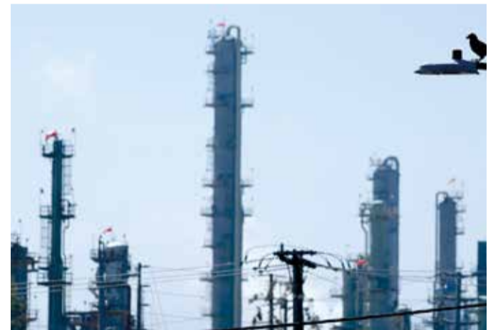
A bird rests on a street light near the Chevron EL Segundo refinery, one of the largest petroleum processing facilities in California
