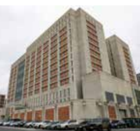
Metropolitan Detention Center (MDC), which is operated by the Federal Bureau of Prisons, is located in Brooklyn, New York
