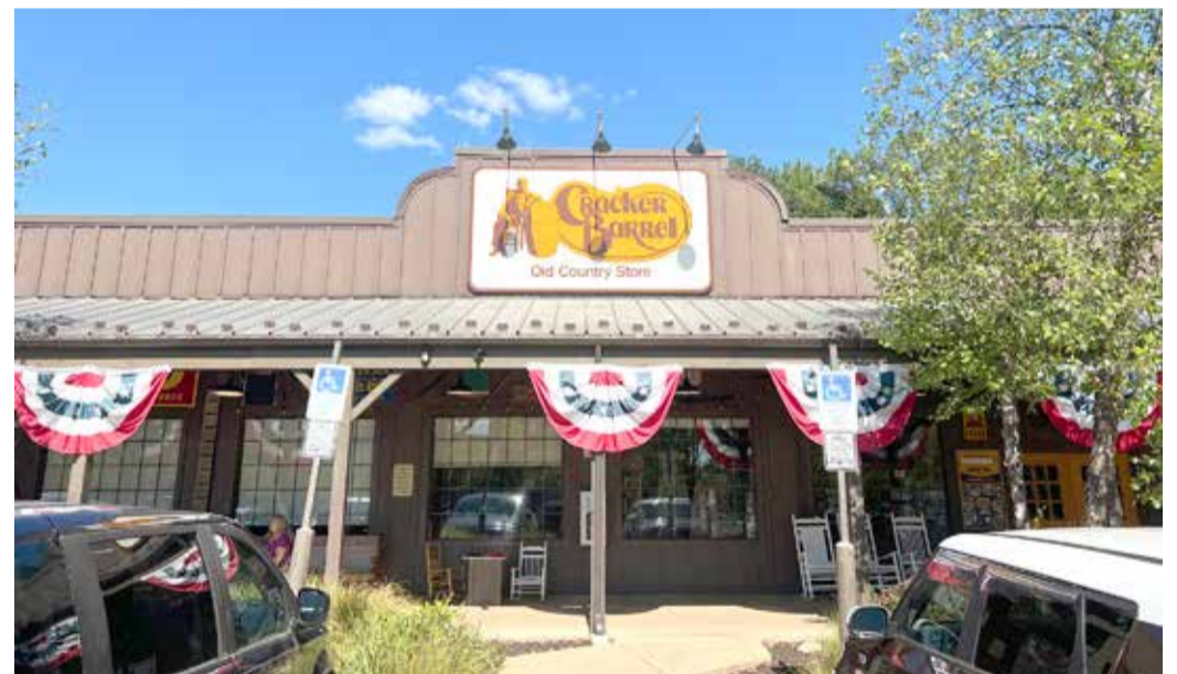
Outside view of the Cracker Barrel Old Country Store in Mount Arlington, New Jersey Washington, United States
