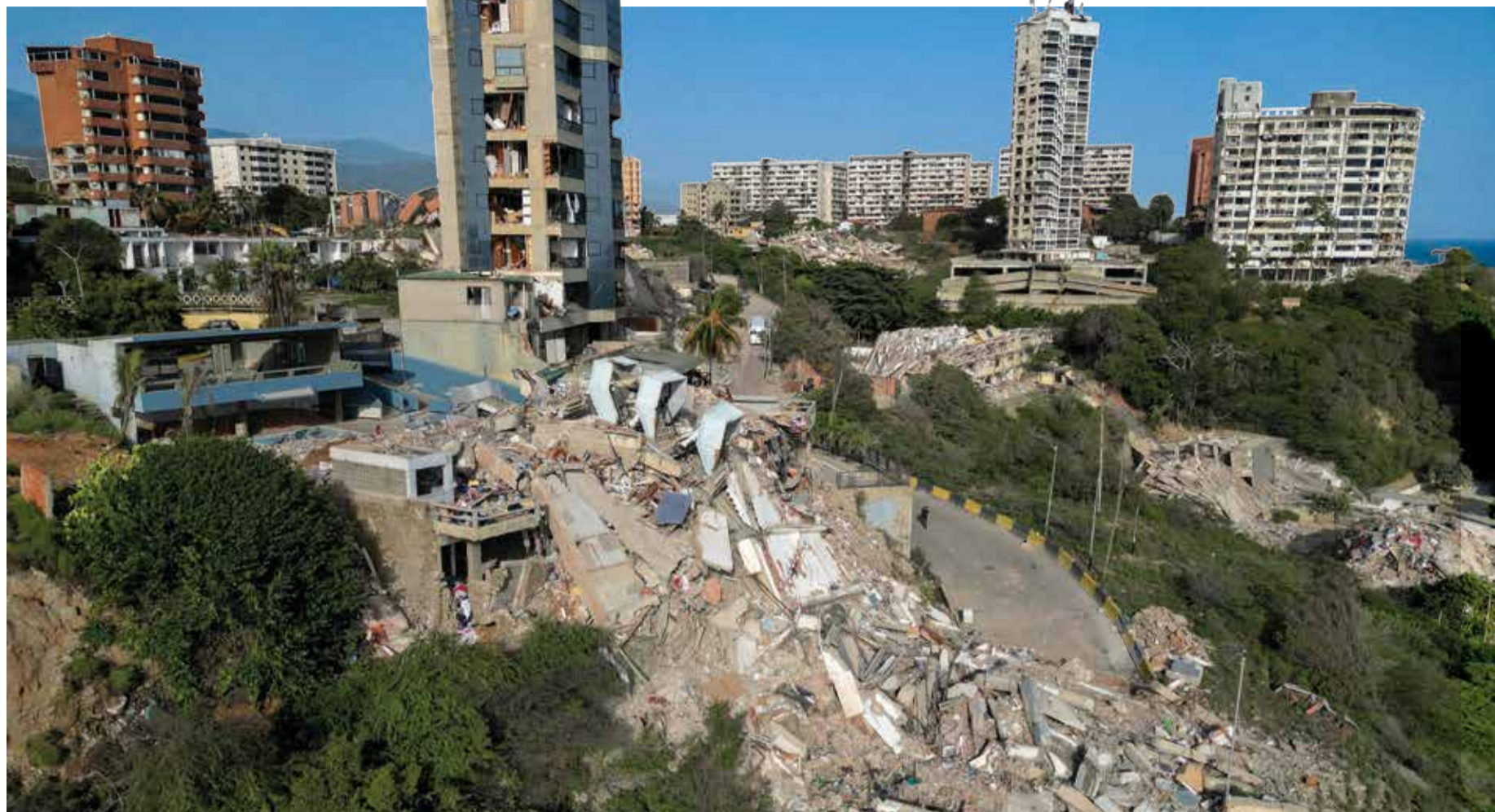
This aerial view shows collapsed buildings in Catia La Mar, La Guaira state, Venezuela
