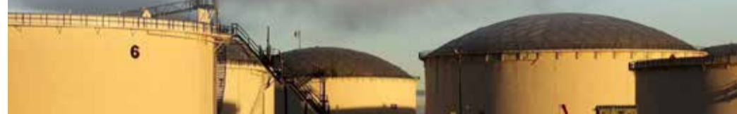
Crude oil storage tanks are seen at the Kinder Morgan terminal in Sherwood Park, near Edmonton, Alberta, Canada
