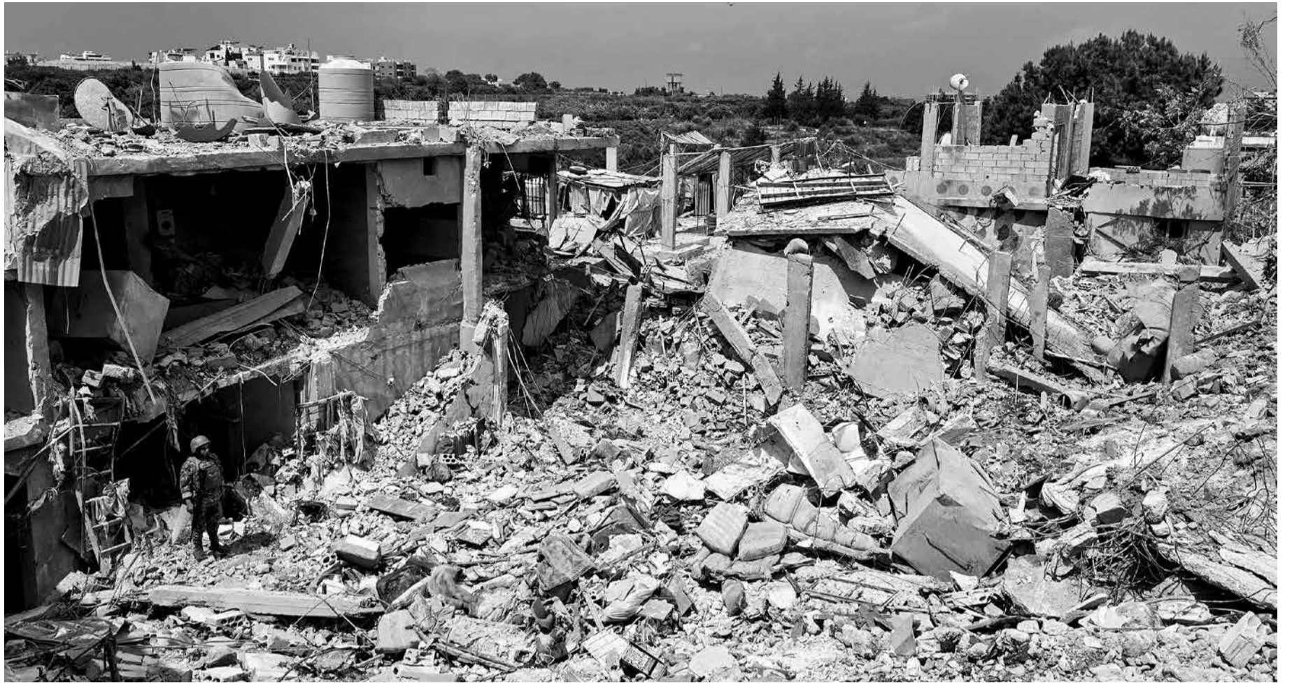
A Lebanese soldier stands on the rubble of a residential building hit the previous day by an Israeli strike near the southern town of Burj al-Shamali
