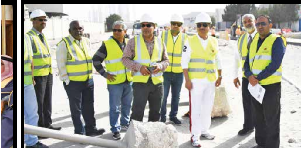
Minister of Works, Municipalities Affairs and Urban Planning Essam Khalaf toured Hidd Industrial Area Roads Revamp Project yesterday. The minister said that the project aims to improve infrastructure in South Hidd (Preparatory Phase), now 86% complete.
