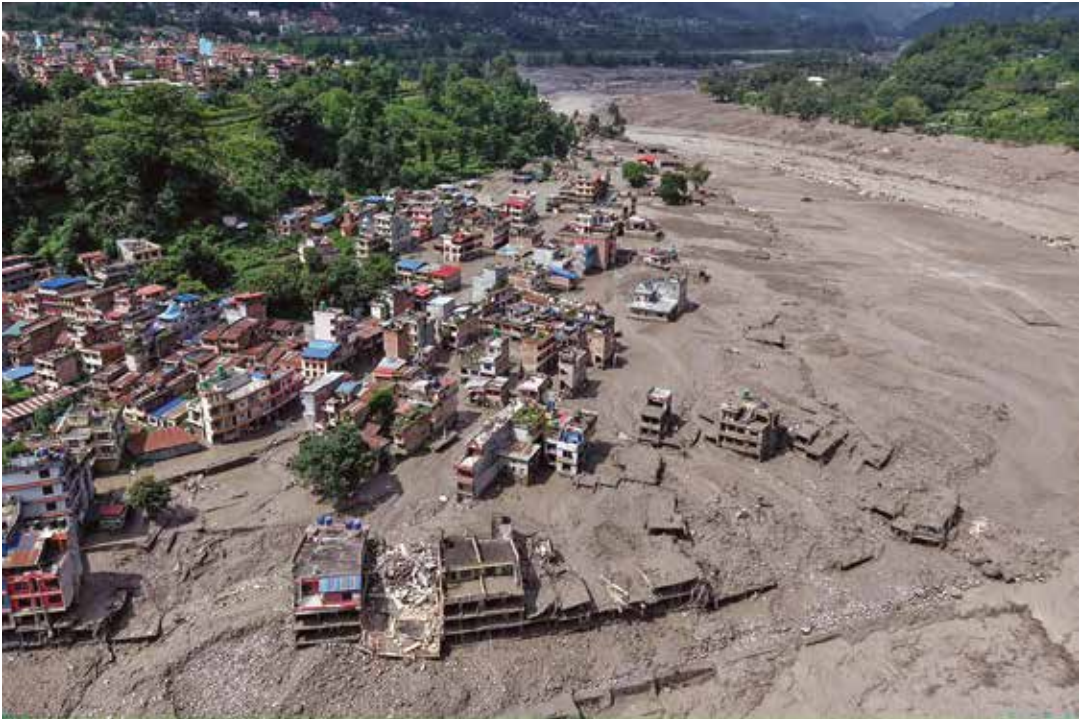
Houses lie partially submerged in muddy water along a riverside after flash floods at Trishuli Bazar in Nepal's Nuwakot district
