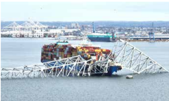
In this aerial image, the steel frame of the Francis Scott Key Bridge sits on top of a container ship after the bridge collapsed, Baltimore, Maryland
