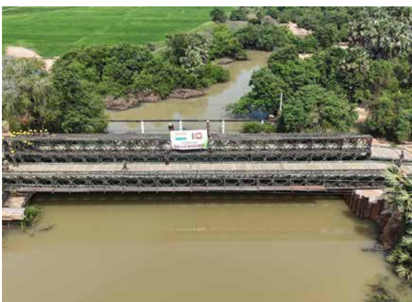
The 120-foot bailey bridge installed by India in Sri Lanka's Kilinochchi District
