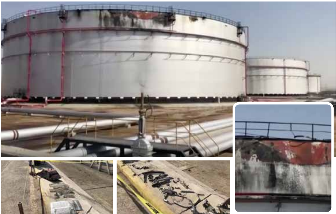
The tank damaged in the attack. Black marks and some damage around its top rim were visible.
