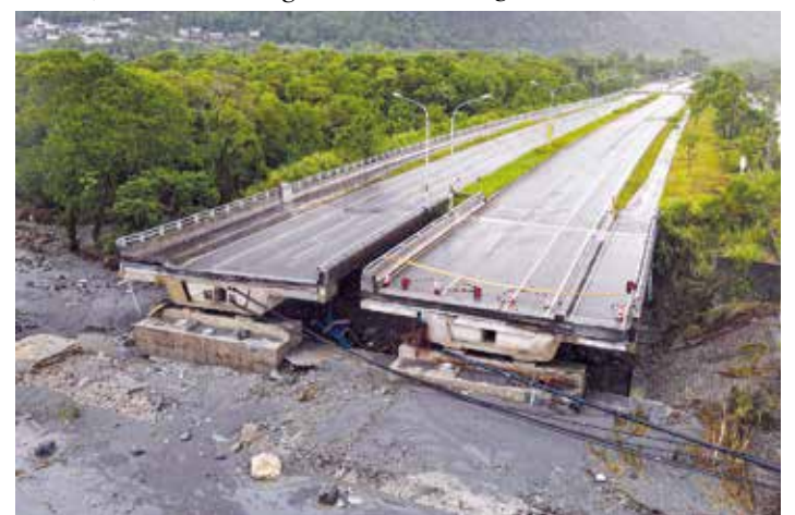
Part of the bridge over Mataian Creek is seen damaged after a barrier lake burst in Hualien
