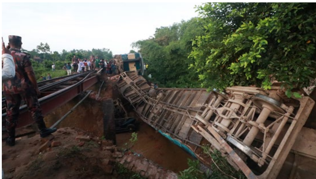
Bangladeshi onlookers gather around a derailed train after a bridge collapse in Kalaura
