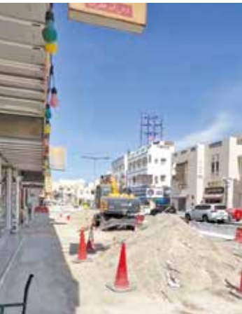
During the removal of the concrete planters
