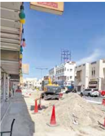
During the removal of the concrete planters
