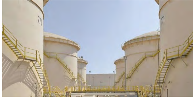
Bapco oil tanks
