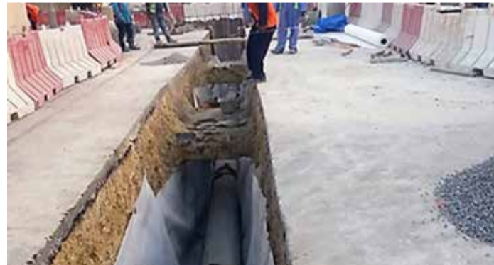
Drainage work in Al Aker
