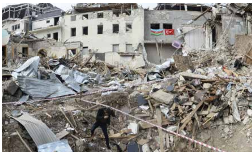
A man walks among the debris of destroyed buildings hit by shelling during the ongoing military conflict between Armenia and Azerbaijan over the breakaway region of Nagorno-Karabakh, in a residential area of the city of Ganja, Azerbaijan
