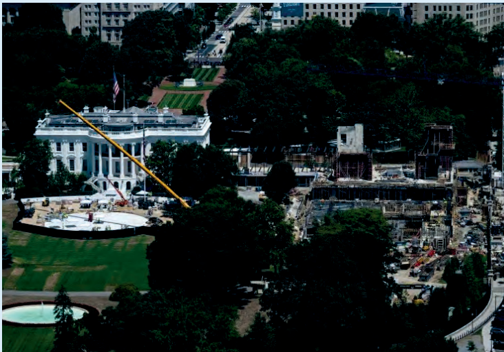
Construction continues on a new helipad on the South Lawn of the White House and the East Wing ballroom
