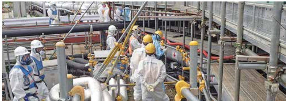
Workers pouring coolant to freeze the underground ice wall around the Fukushima Daiichi nuclear power plants in Okuma, Fukushima
