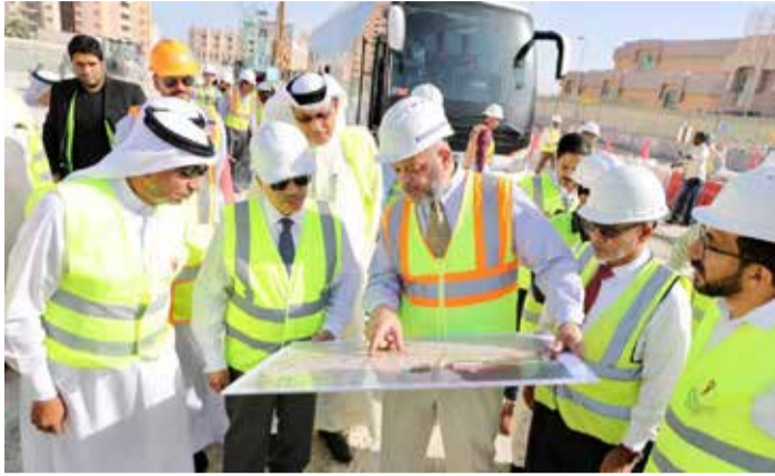
Eng. Khalaf is briefed on the project's progress as excavation work goes full blast
