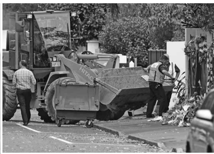
A digger delivers a load of gravel to the Al Noor mosque in Christchurch
