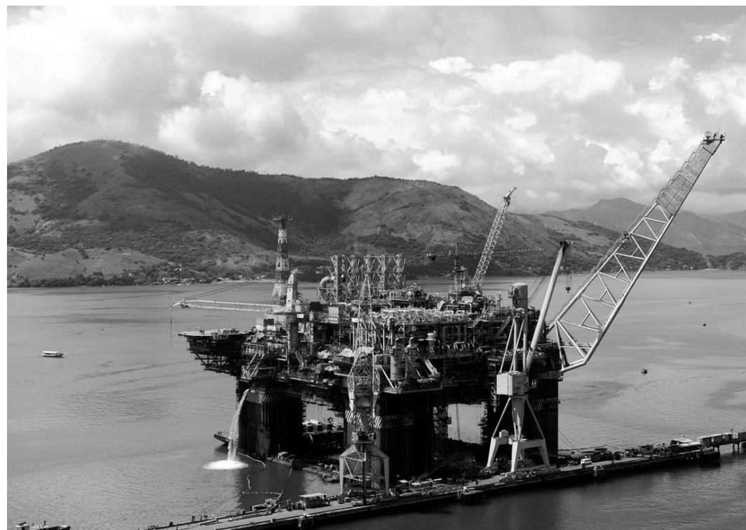
Petrobras pumps 500,000 barrels of oil a day from pre-salt fields. Pictured, assembling a new oil platform (Courtesy of Reuters)
