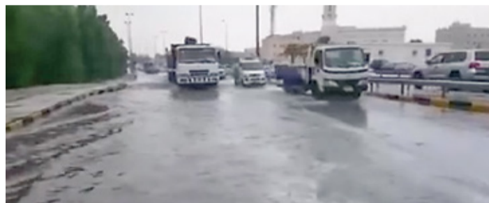
Vehicles wade through flooded roads in Riffa.
