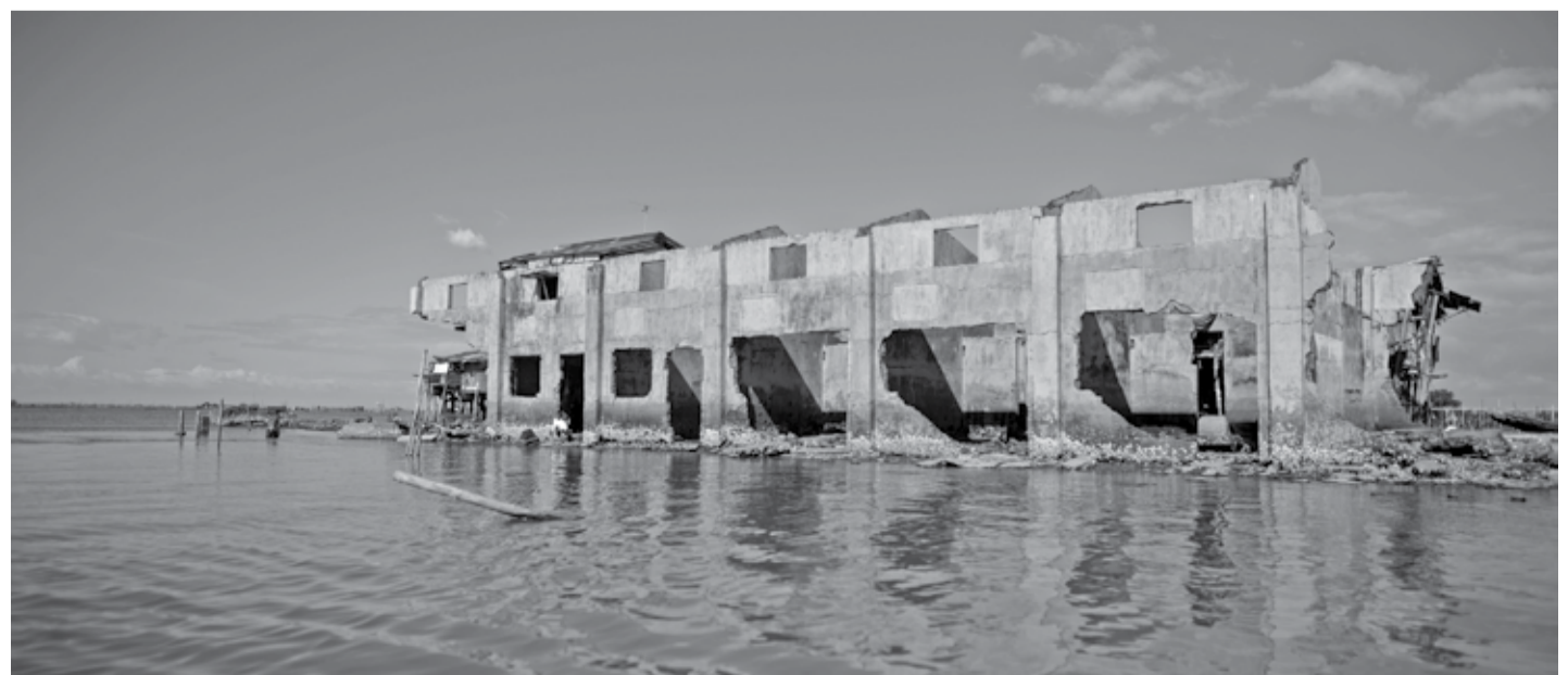
An abandoned structure amid encroaching bay waters in Sitio Pariahan, Bulacan
