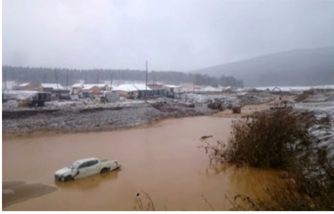
Investigators said they opened a criminal probe into the violation of safety rules after the collapse of a dam in Siberia
