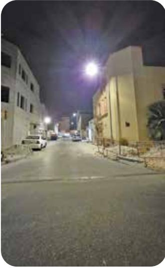
One of the streets in A'ali where lighting was recently installed.
