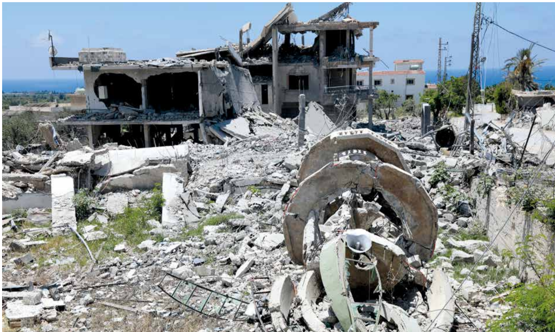
The site of an Israeli attack that destroyed houses and carpentry shops in the village of Al-Qailah in the Tyre district in southern Lebanon
