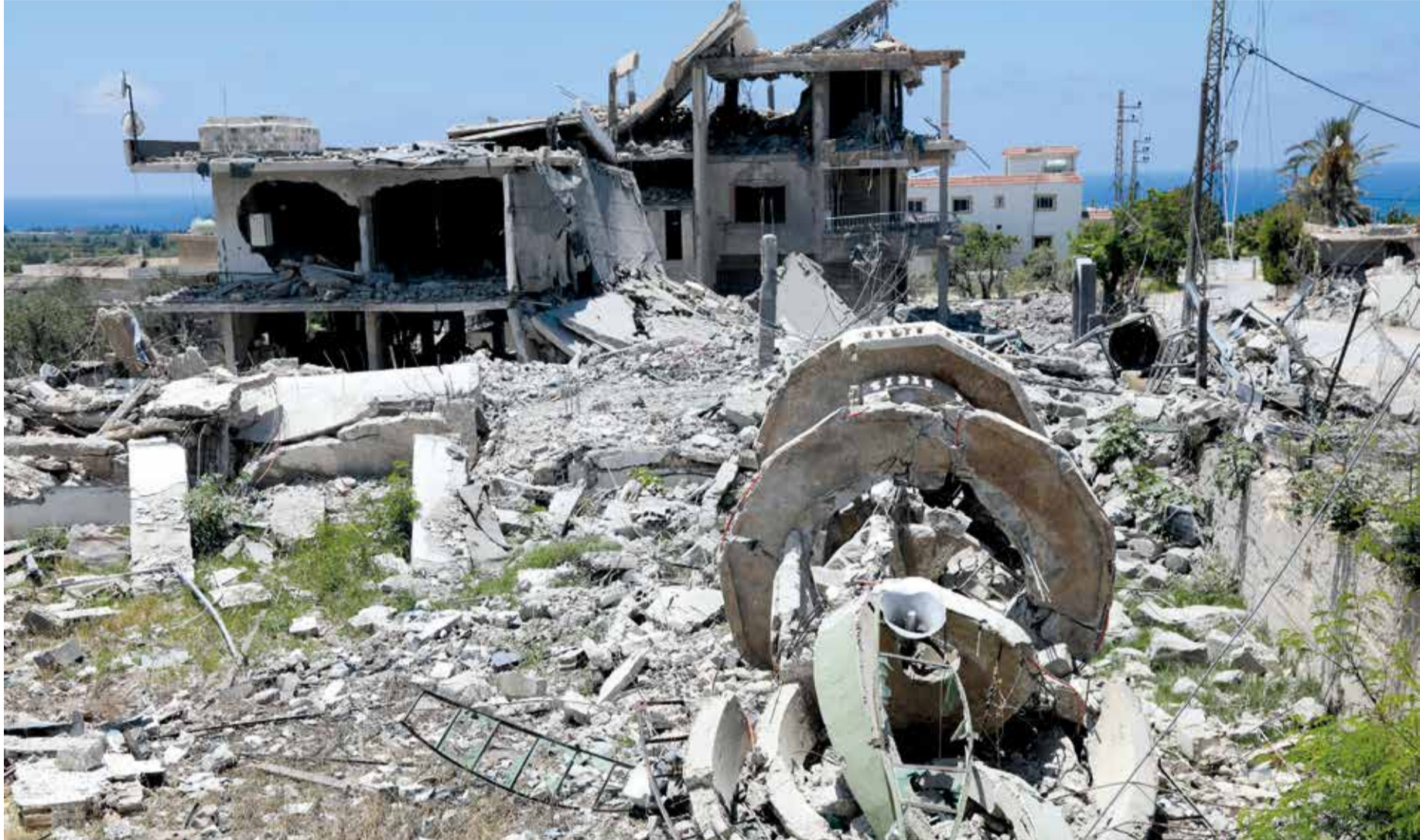
The site of an Israeli attack that destroyed houses and carpentry shops in the village of Al-Qlailah in the Tyre district in southern Lebanon
