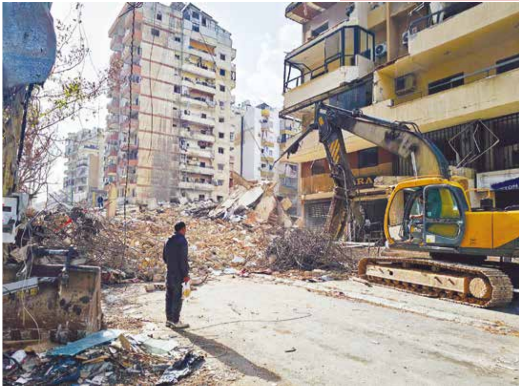
A bulldozer clears the rubble from the site of an Israeli airstrike as people return to Beirut's southern suburbs
