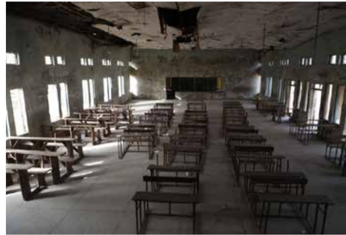
Empty classroom of the Government Science College where gunmen kidnapped dozens of students and staff, in Kagara
