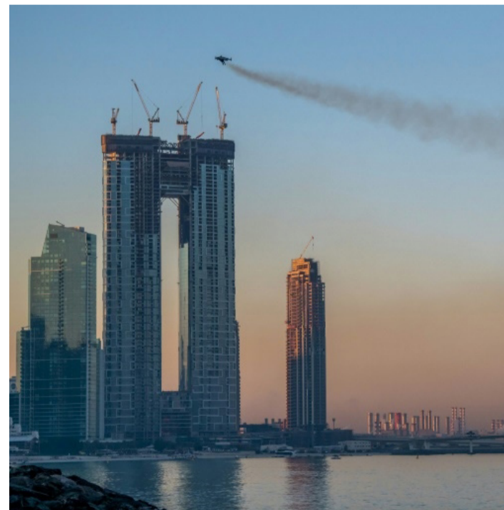
Reffet soared to heights of up to 1,800 metres (nearly 6,000 feet) over the skyscrapers of Dubai
