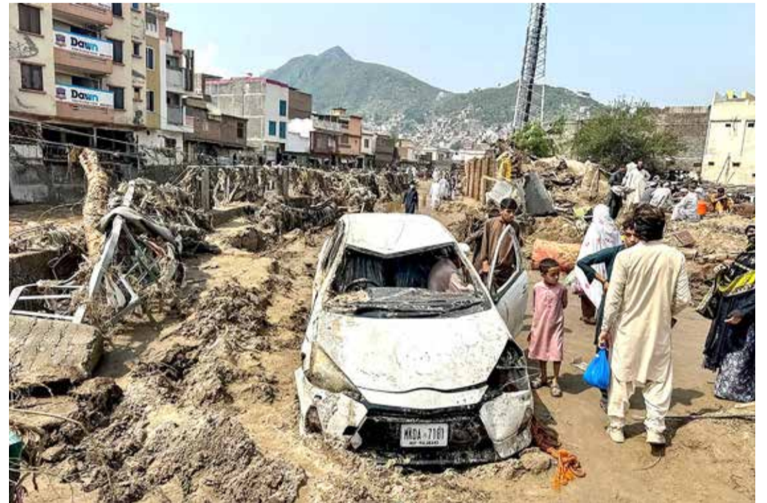
People gather near a damaged vehicle and scattered debris after the road washed out following a flash flood in Mingora, the main city of Swat Valley, in monsoon-hit northern Pakistan's mountainous Khyber Pakhtunkhwa province
