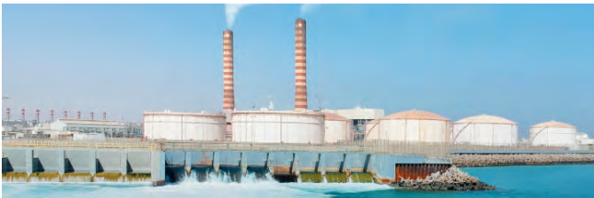
Reports indicate that the Zour Thermal Power Plant in Kuwait suffered damage to power generation units following an attack on July 17, 2026.
