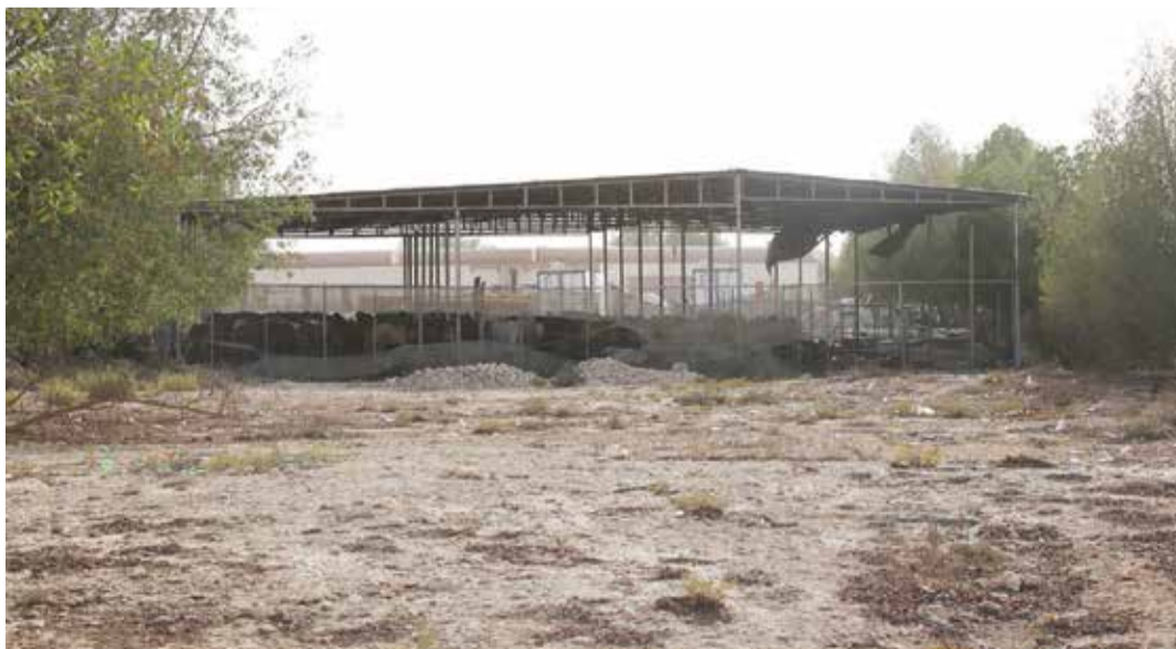
Despite several notices, the slaughterhouse continues to function in the village.
