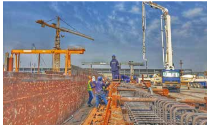
Construction work in progress
