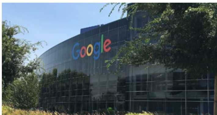
The Googleplex is the corporate headquarters complex of Google and its parent company Alphabet Inc. It is located at 1600 Amphitheatre Parkway in Mountain View, California, United States.
