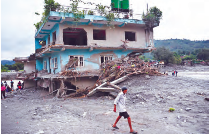
A man walks past a damaged house covered in sludge in the aftermath of flash floods at Devighat in Nepal's Nuwakot district
