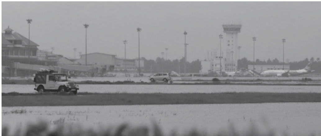
Kochi's International airport apron is seen flooded following monsoon rains
