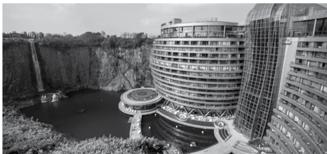
The InterContinental Shanghai Wonderland, built inside a formerly abandoned quarry, about 32 kms (20 miles) southwest of Shanghai
